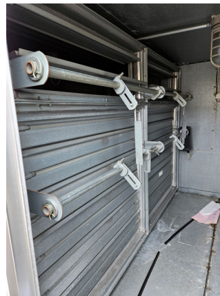
Left: the min/max OA damper assembly; Right: the inclinometer (a tilt sensor) installed on the return air damper
