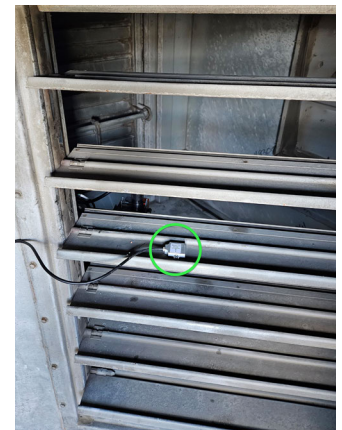
Left: the min/max OA damper assembly; Right: the inclinometer (a tilt sensor) installed on the return air damper
