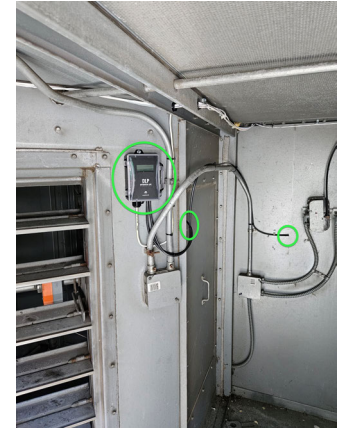
Left: velocity probes installed at the supply air fan inlet Right: pressure assist sensor on the return air damper
